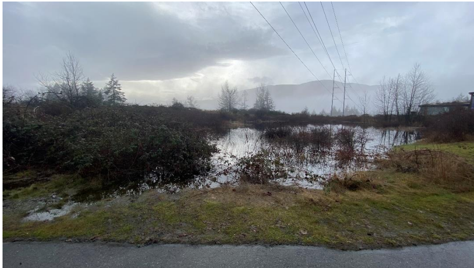
Photo 23. Jan. 13, 2023. Looking west at the ditched outlet of the constructed pond adjacent to the Tourism Nanaimo Visitor Centre following a significant rainfall event.
